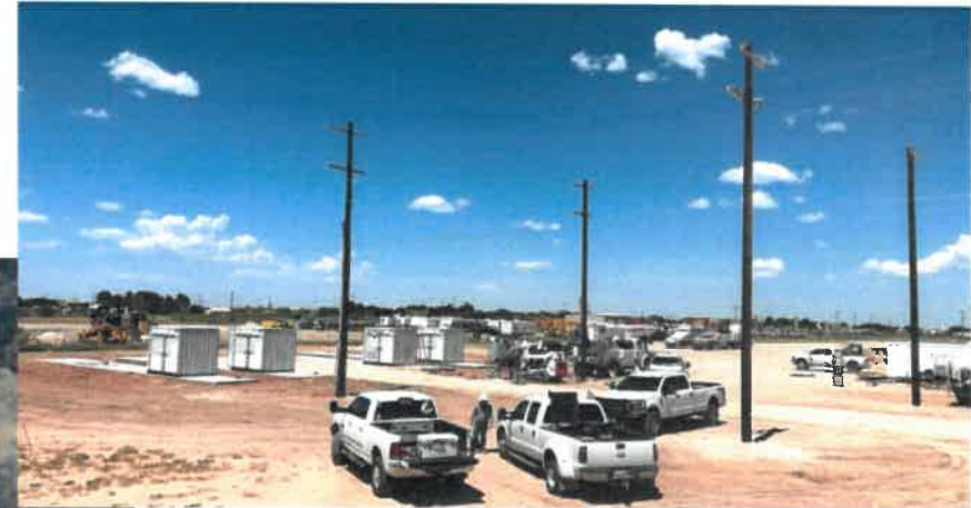
BRP Project in Construction in Odessa – footprint: ½ acre
